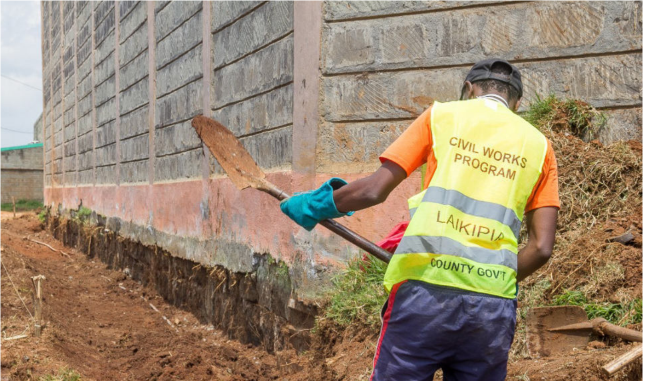
Youth working on a road in Nyahururu under the civil works programme of county government of Laikipia
